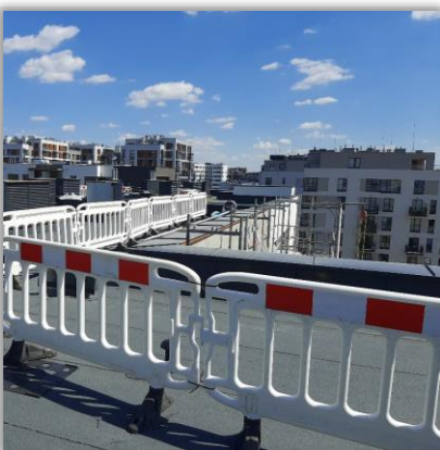
Fencing the danger zone on the roof Woronicza/Suwak R4R
