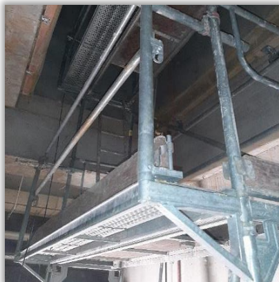
Scaffolding in the installation shaft Esencja
