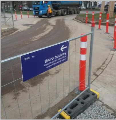
Securing the entrance for trucks and directing traffic MidPoint 71
