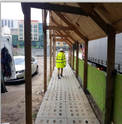
Protective roof for visitors REACT
