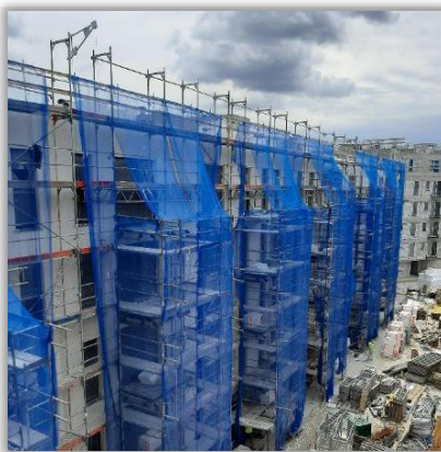
Elevated scaffolding to secure the works on the roof Esencja
